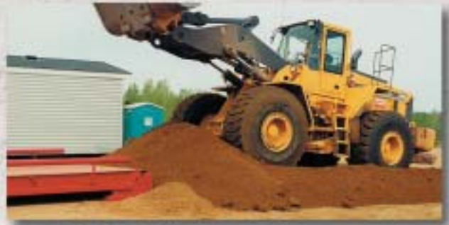
2. Backfill to bulkheads and finish ramps.
